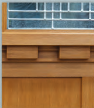
Details of the Craftsman Fir Grain Construction
